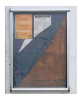
The material cannot be tacked to the back of the board, as the board cannot be removed from the frame. A temporary solution has been offered by Monmouth Fabrics (tacking the material to the edge of the board with heavy duty tacks). This solution, however, is unlikely to resolve the issue long-term.
